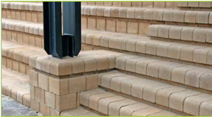
CLOSE UP OF BLOCKS CUT TO SHAPE
