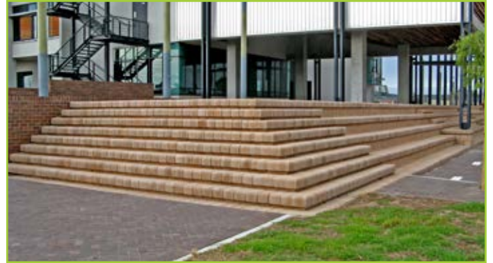
STAIRWAY AND RAMP COMBINATION
